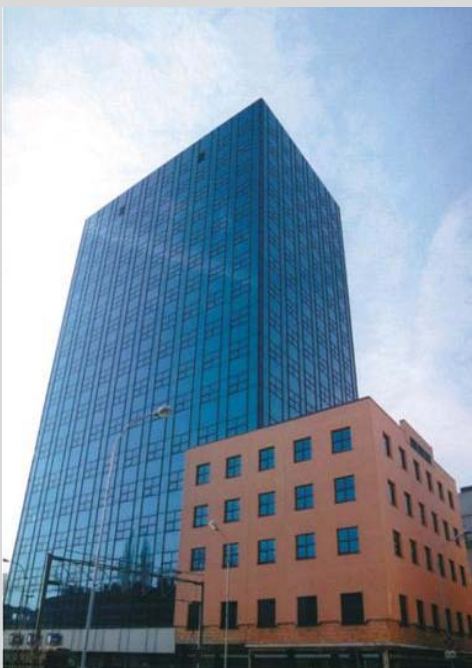
PHILIPS SHARED SERVICES CENTRE, ORION BUILDING, ŁÓDŹ
